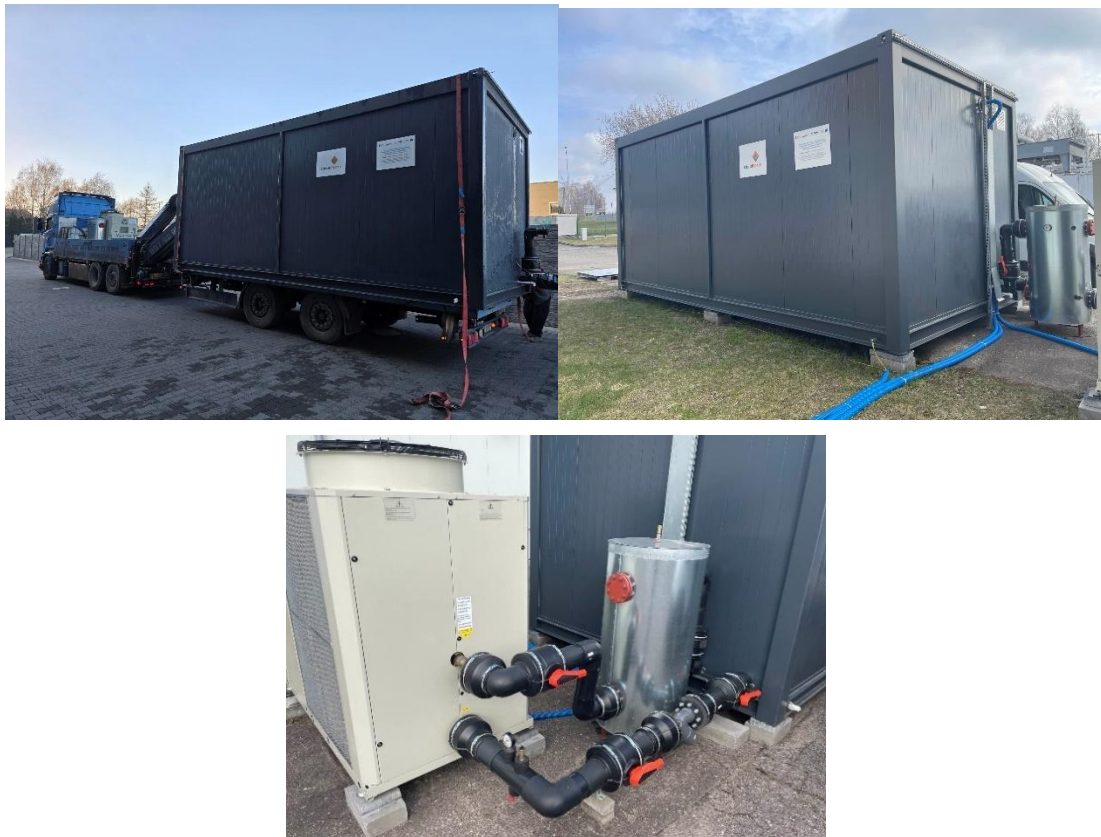
Figure 129. Pilot 2 Container and chiller relocation to Łódź, CF location
